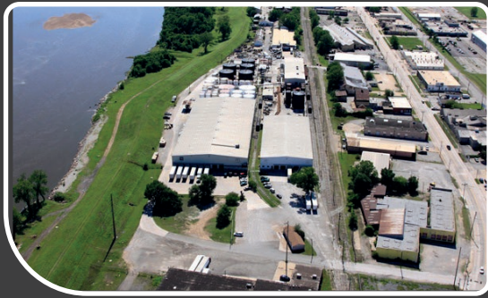
Grease Lubricant Plant Tulsa, Oklahoma
